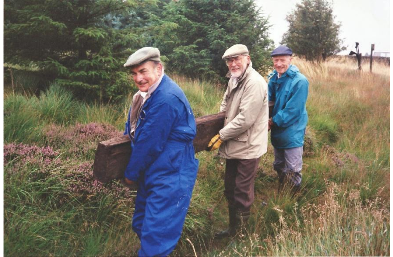
Colin Newton, Roger Stark, Jack repairing bridge at Norwood Edge
