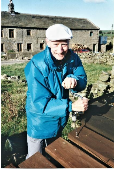
Jack repairing bridge at Bankfoot Farm
